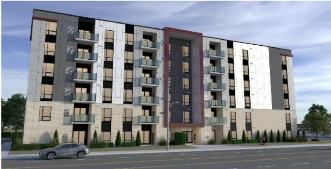
NORTH ELEVATION - FACING TECUMSEH ROAD
